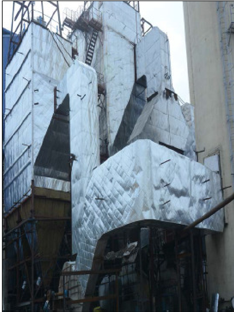
ESP for 20 & 90 TPH Boiler Capacity
